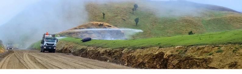
Having originally priced the project in October 2019, Covid lockdowns delayed project commencement until June 2021. Since our first establishment in 2021, we have completed over 1,100,000m2 of hydro mulch and Soil Blanket, as we stabilized and revegetated dumpsites, cut batters, sediment ponds, fill sites, and various earthworks areas throughout the project.
