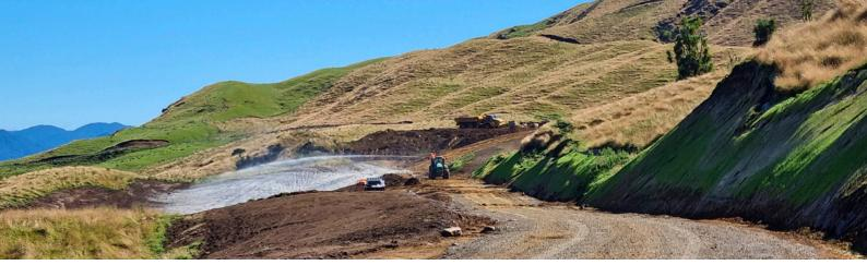
Being able to stabilize areas with the cannons on our trucks meant we could reach up to 100 meters horizontally and 45 meters vertically from the truck, without having to run hoses or have staff members working on uneven ground. For the large cuts, we were able to revegetate all of these with our cannons, whereas other hydroseed contractors would have needed knuckle booms or similar to access the top of these cuts.
