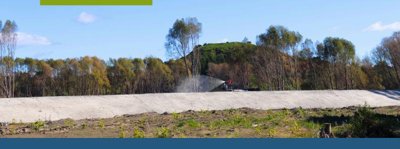
At one of the Puketapu sites, the earthworks contractor was working overtime to topsoil the stop bank before a rain event came through. They finished the 2ha site just in time and we were able to Hydro Mulch the entire 2ha in one day on site with our 8x8 and T400 (the largest hydro mulcher in New Zealand). After the rain event, the stop bank had no sediment run off, with no rework required. Within 4 weeks we achieved an 80% grass strike, and local residents could move back into their homes.
